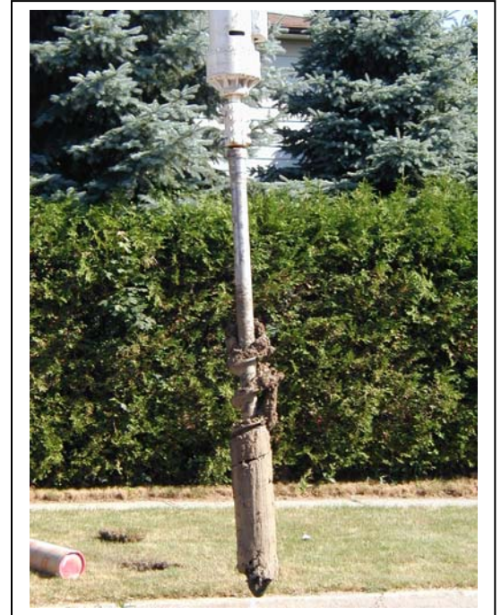
Auger Excavation
